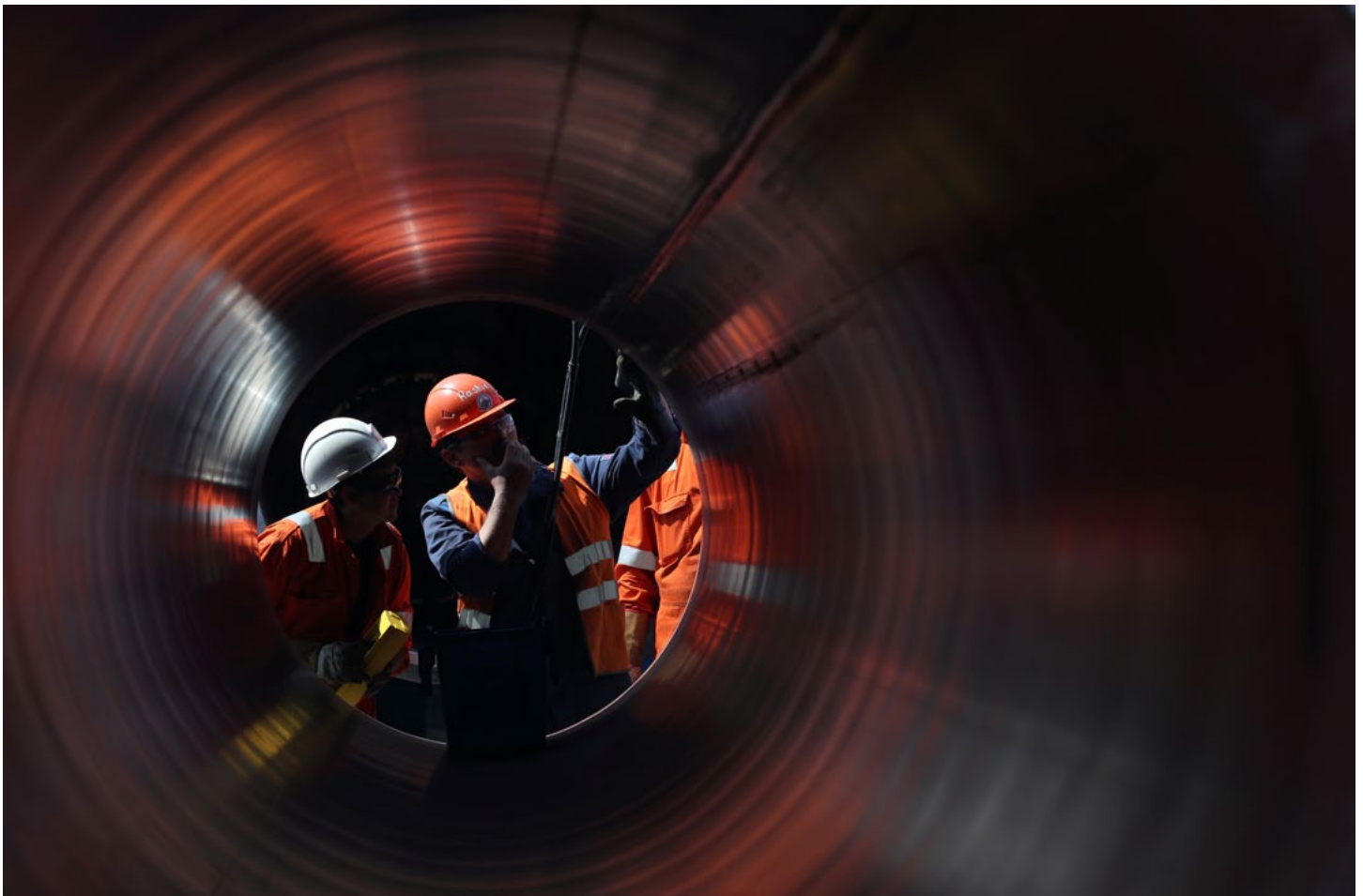
Workers are seen through a pipe at the construction site of the Nord Stream 2 gas pipeline, near the town of Kingisepp, Leningrad region, Russia, June 5, 2019. REUTERS/Anton Vaganov.
