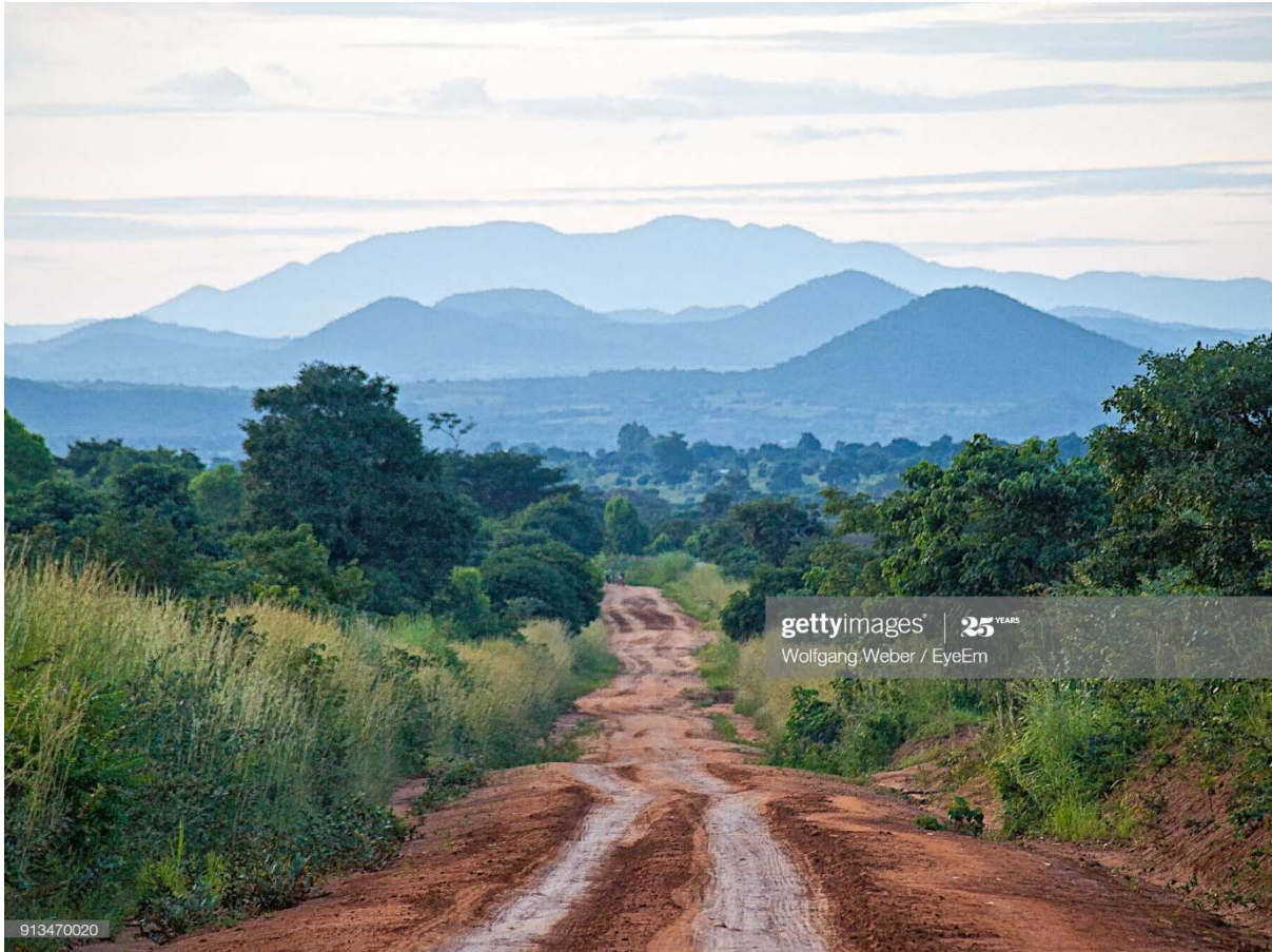
Figure 1. Unpaved road providing essential market access to farmers and consumers. Roads like these linking villages and cities to boarder points can stretch for hundreds of kilometres and can turn non-operational during the rainy season.
